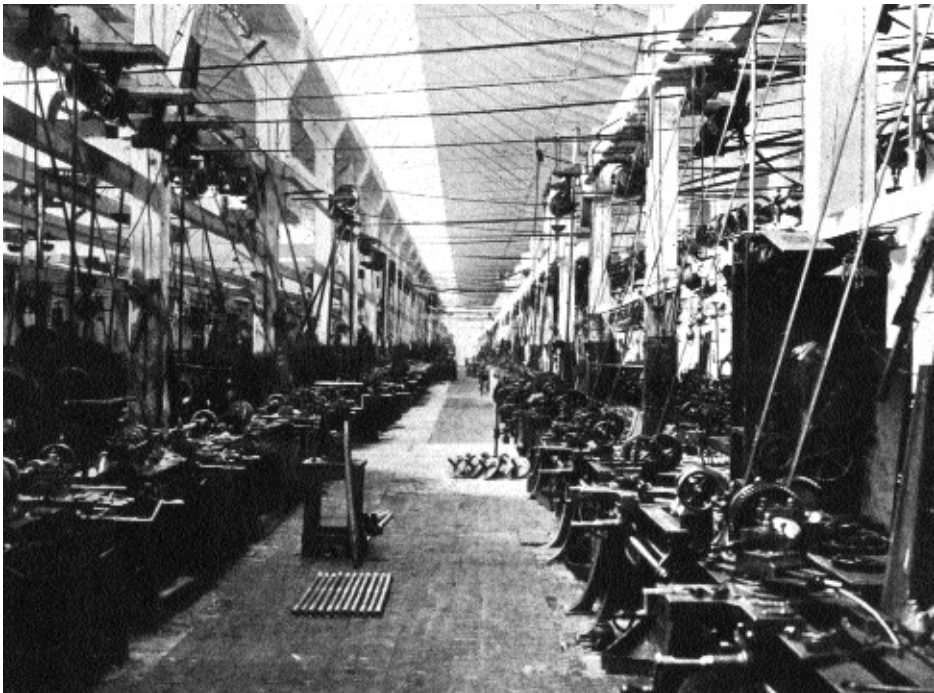
End view of No. 2 bay, looking east
