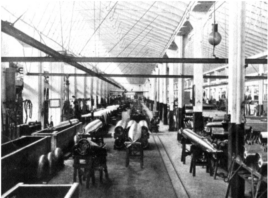
View of No. 3 bay, looking east
