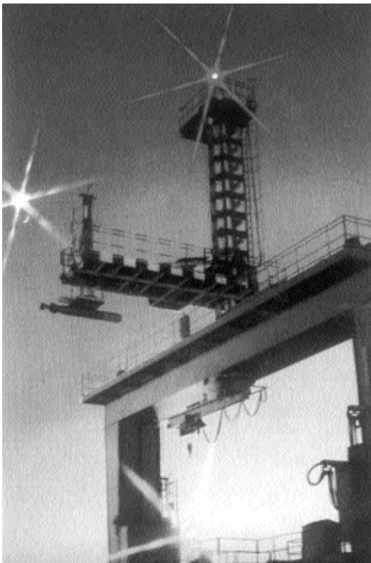
Fig. 65: Salviano (Livorno). Bridge-crane used for torpedo tests in pool (simulation of helicopter launches and other) (Since 1984) (WASS Historical Archive).
