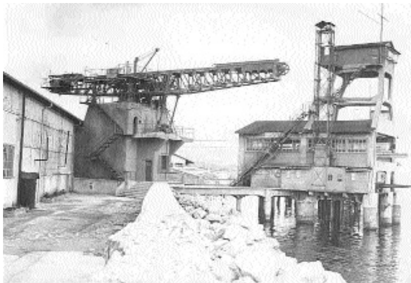
Fig. 28: Catapult suitable to simulate stresses present in a torpedo launched from aeroplanes. To the right the Giuseppe Orlando launching station (1933-1934) (WASS Historical Archive).
