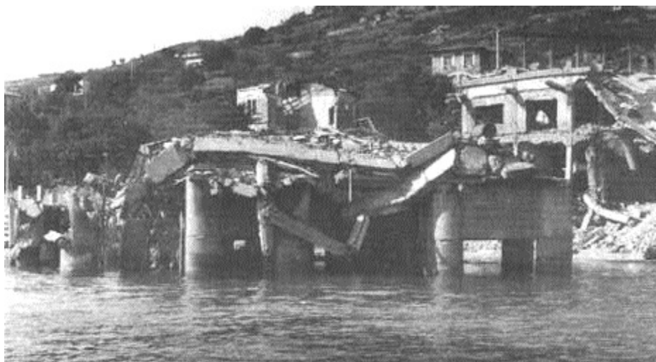
Fig. 42: Porto Santo Stefano. Effects of allied bombing and german mining on the torpedo launching station (1943-1945) (WASS Historical Archive).
