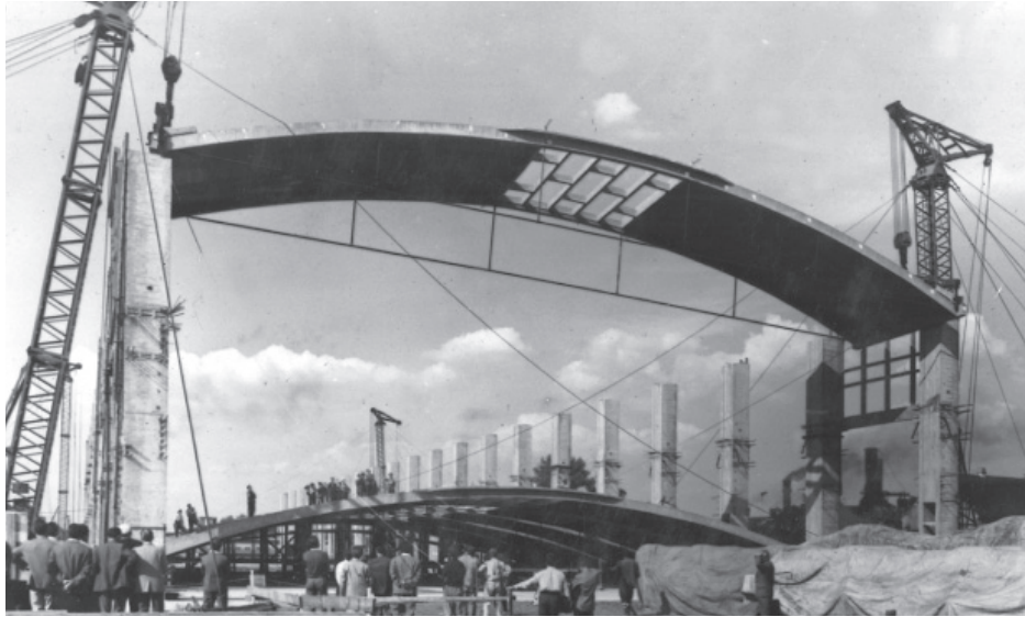
■ Illustration 13. Cable factory Budapest XI. 1962, Mátrai, Pászti, lifting the roof element
