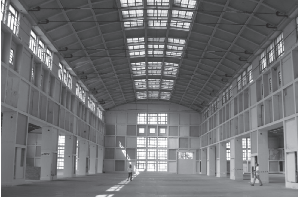
■ Illustration 14. Ikarusz autobus factory Budapest XVI. 1958-59, Mátrai, Pászti, picture inside the hall in 2013
