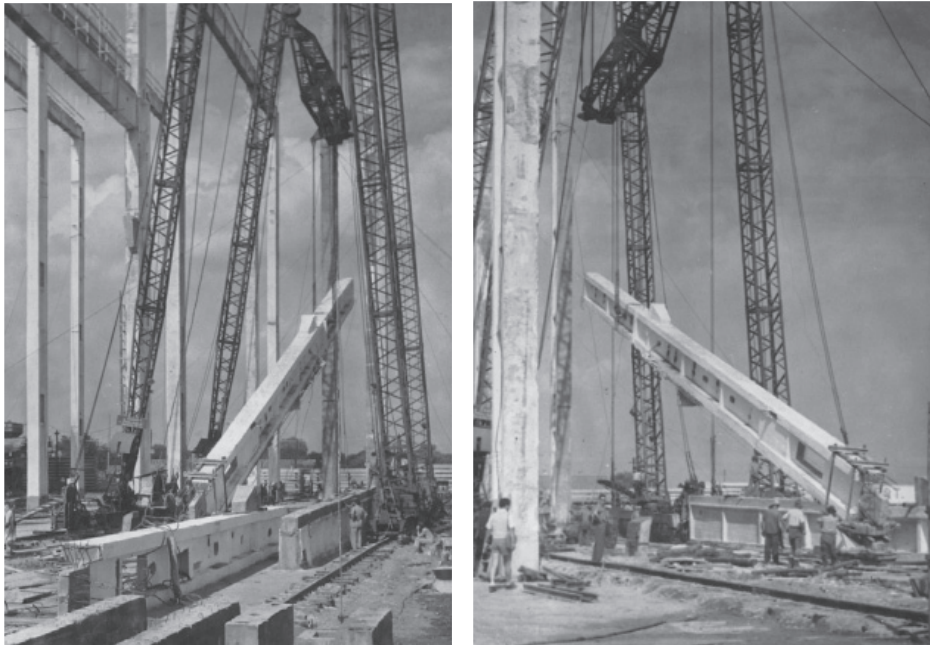
■ Illustration 3-4. Berente power plant, 1953, Gy. Mátrai, K. Pászti lifting the load bearing pillar element
