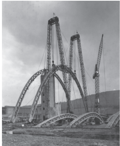
■ Illustration 9-10. Chemical manure storage, Kazinbarcika, 1949-52, Gnädig, lifting the trussed main girder
