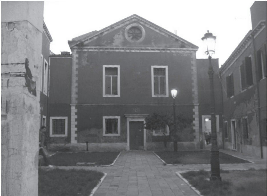
■ Figure 1. Ex- St. Anne cloister, the headquarter of the Marine Collegium during the period 1811-1848
